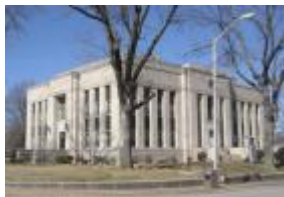
Obion County Courthouse
