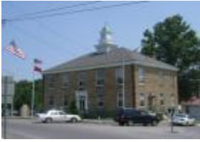
Pickett County Courthouse
