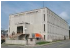
Union County Courthouse
