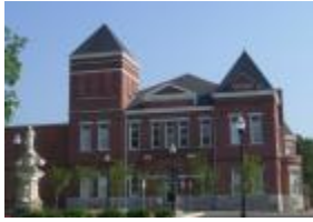
Warren County Courthouse
