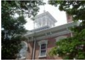
Coffee County Courthouse
