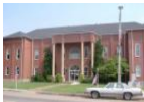
Bledsoe County Courthouse
