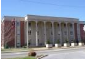
Anderson County Courthouse
