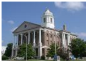
Bedford County Courthouse
