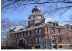
Henry County Courthouse
