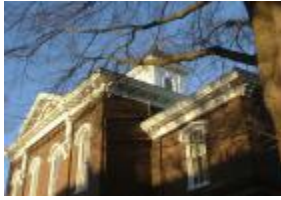
Loudon County Courthouse
