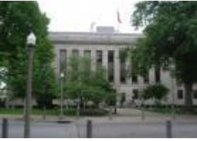
Madison County Courthouse
