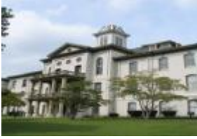
Hamblen County Courthouse
