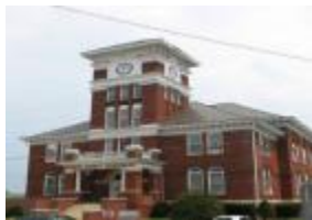
Monroe County Courthouse
