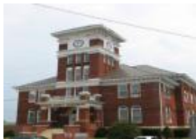
Monroe County Courthouse
